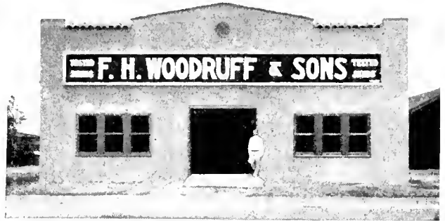
Above: This warehouse at Mercedes, Texas, serves the Lower Rio Grande Valley and Teaxs.
